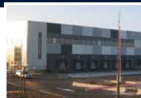
SPI LOGISTICS Saint-Quentin-Fallavier Location : 30 000 m 2
